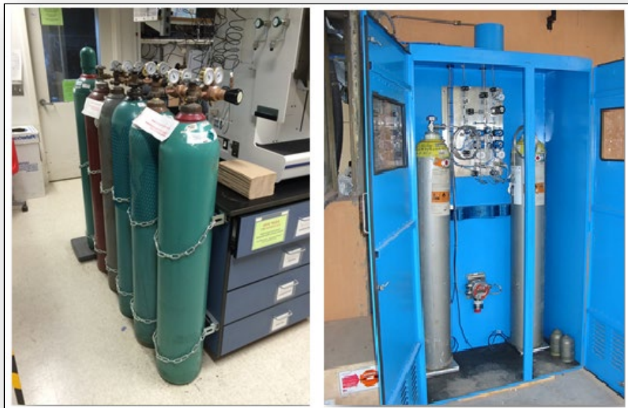
Figure 3.15: Gas Cylinder Storage
